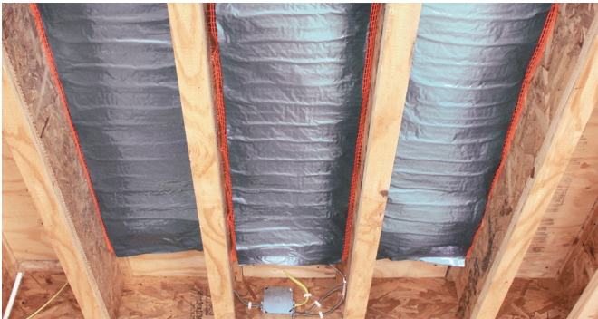
SunTouch UnderFloor - multiple joist bays
